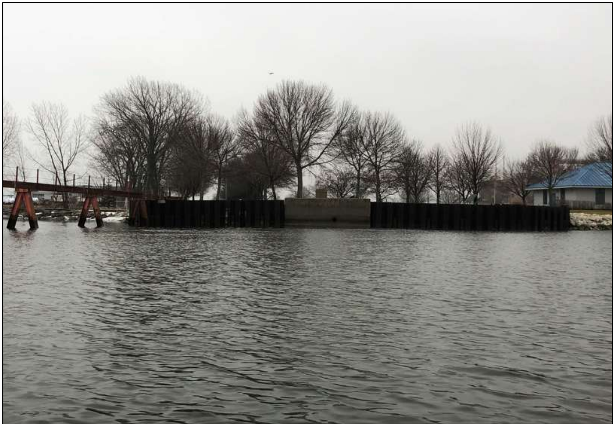
Figure 3-1. View of the GBF Outfall (Concrete Shorewall).
