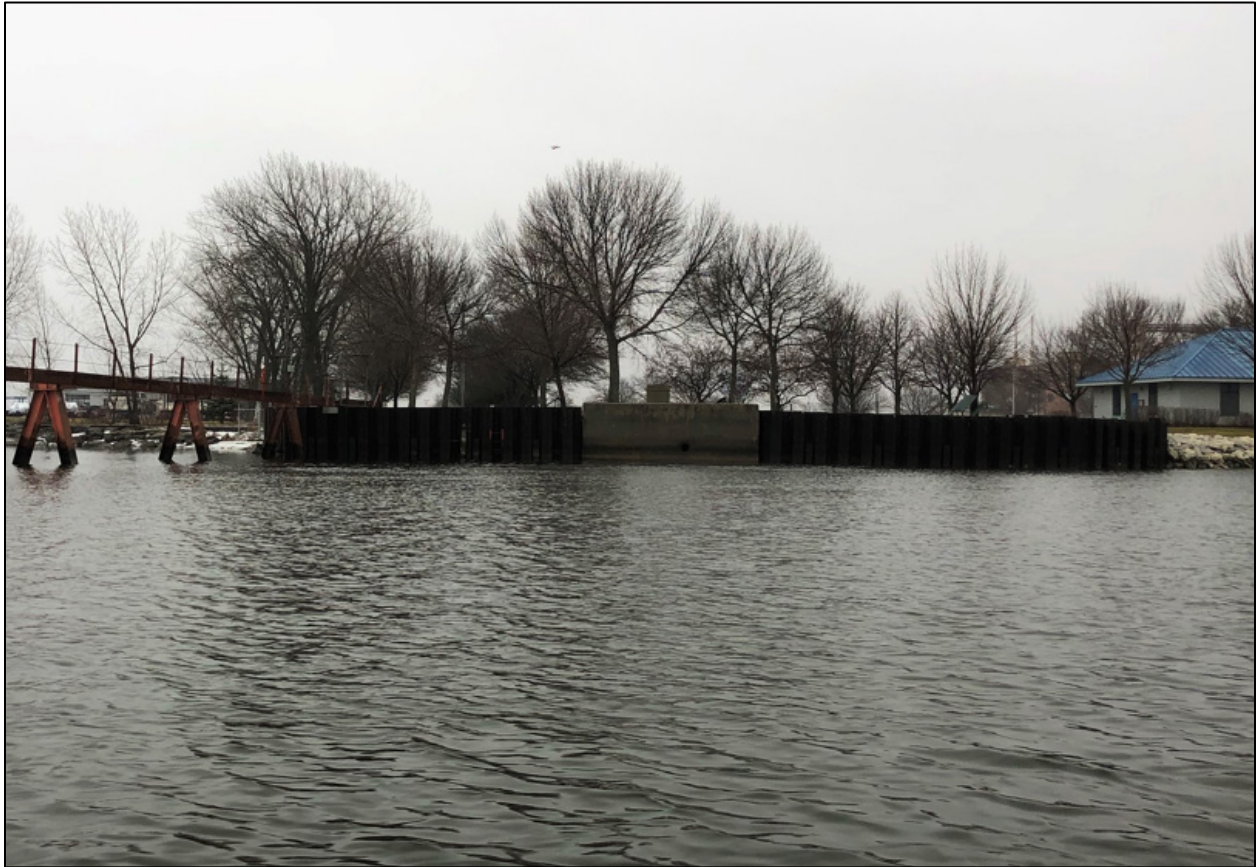
Figure 3-1. View of the GBF Outfall (Concrete Shorewall)
