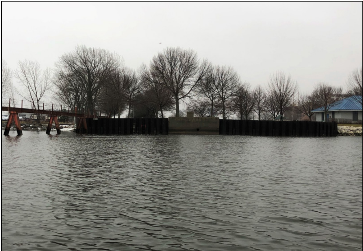
Figure 3-1. View of the GBF Outfall (Concrete Shorewall)
