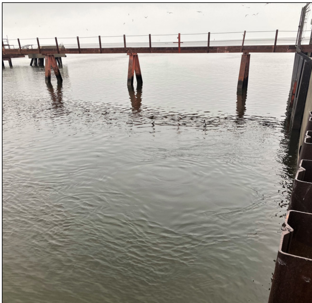
Figure 3-2. Visible Swirling/Roiling in the Fox River Above the GBF Outfall (Outfall is Concrete Structure at Right)
