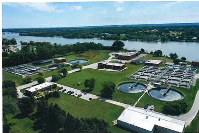
An aerial view of NEW Water's De Pere Facility.
