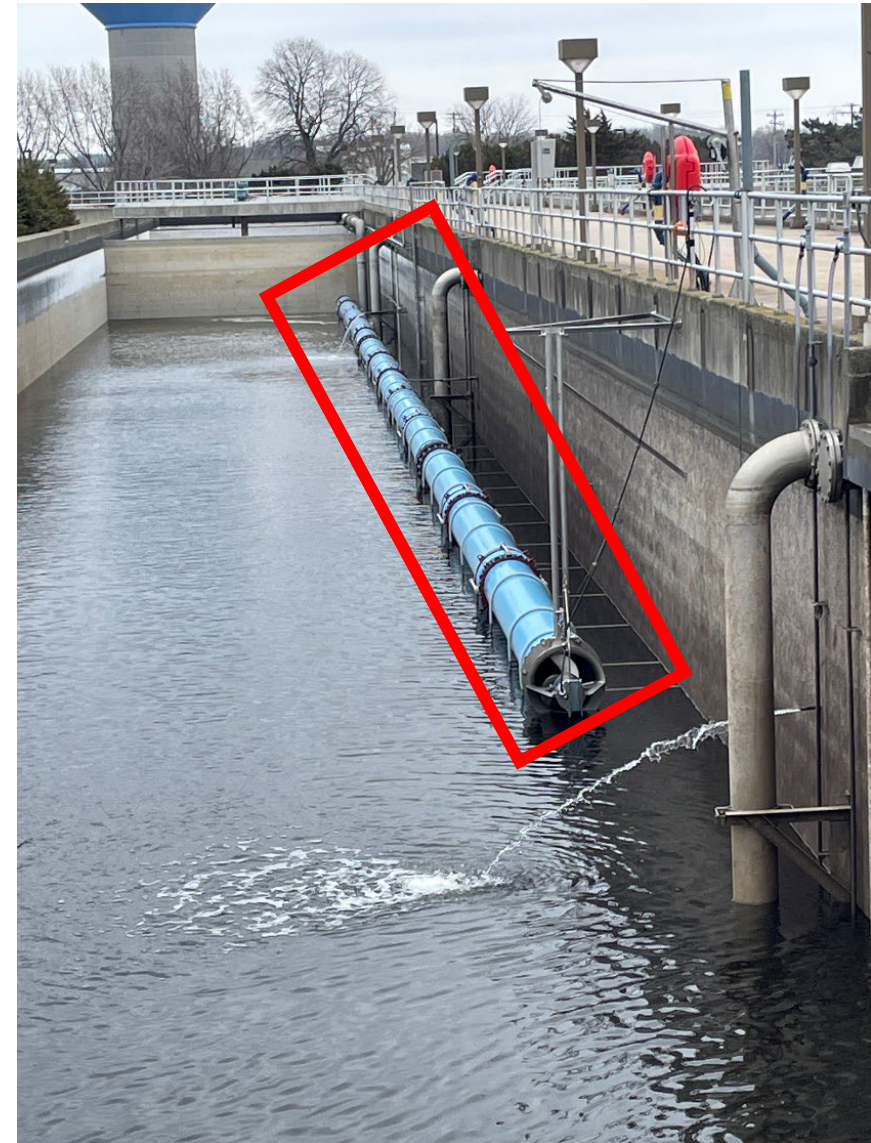
Mixed Liquor Recycle Pump
