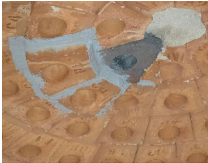
Figure 3 FBI Dome Castable Repair
