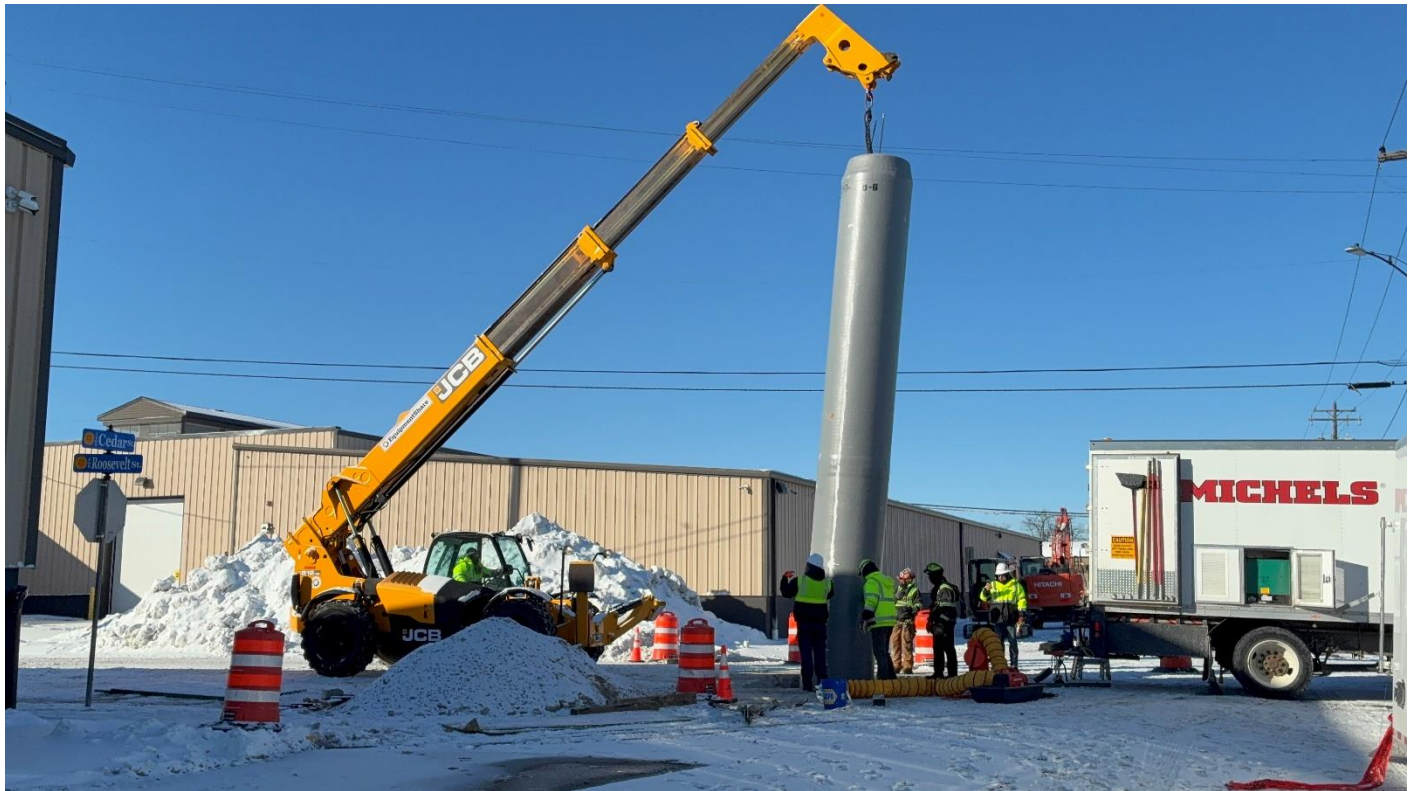
Photo 1 – Michels installing the FRP manhole insert on Roosevelt Street.
