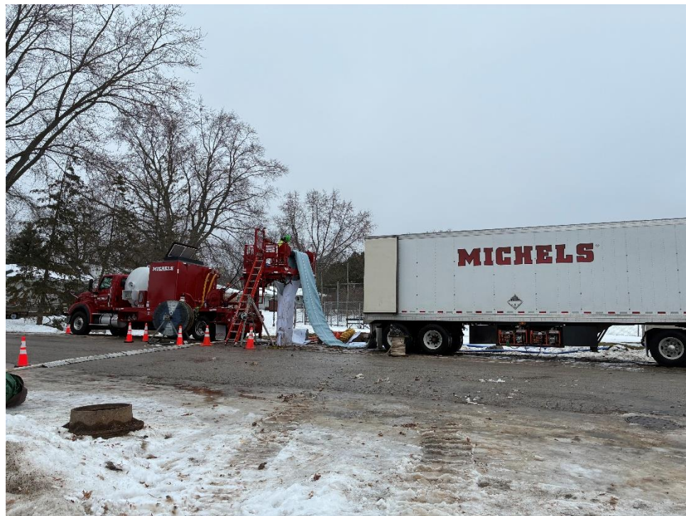
Photo 2 – Michels installing 30" CIPP liner segment at Emilie Street.
