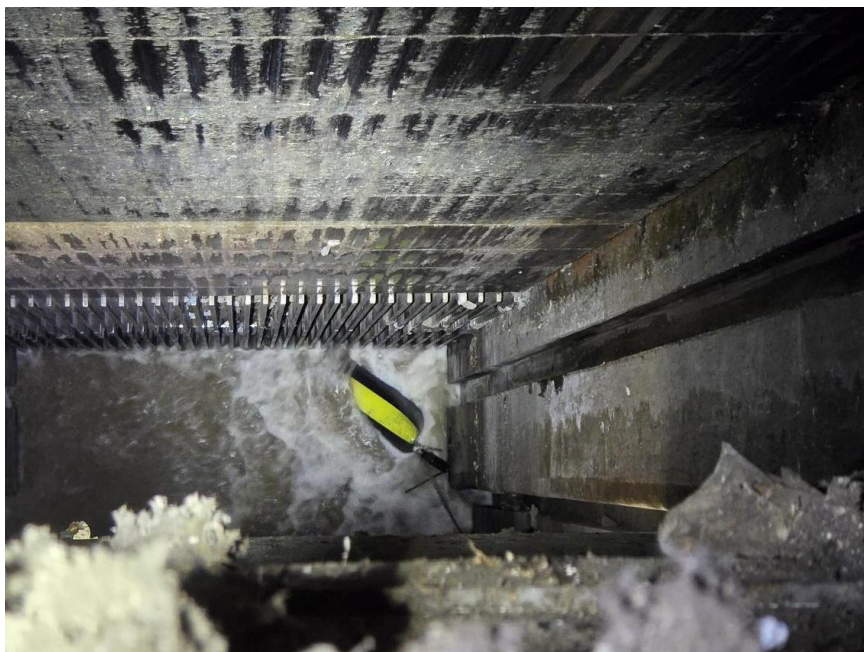
Photo 2 – ECI attempting to retrieve the sewer plug from the pump station wet well.
