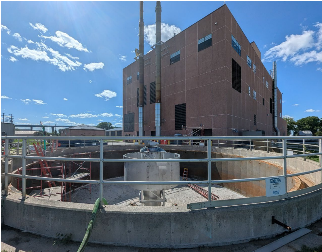
Figure 1: Progress Towards Installation of Gravity Thickener #4
