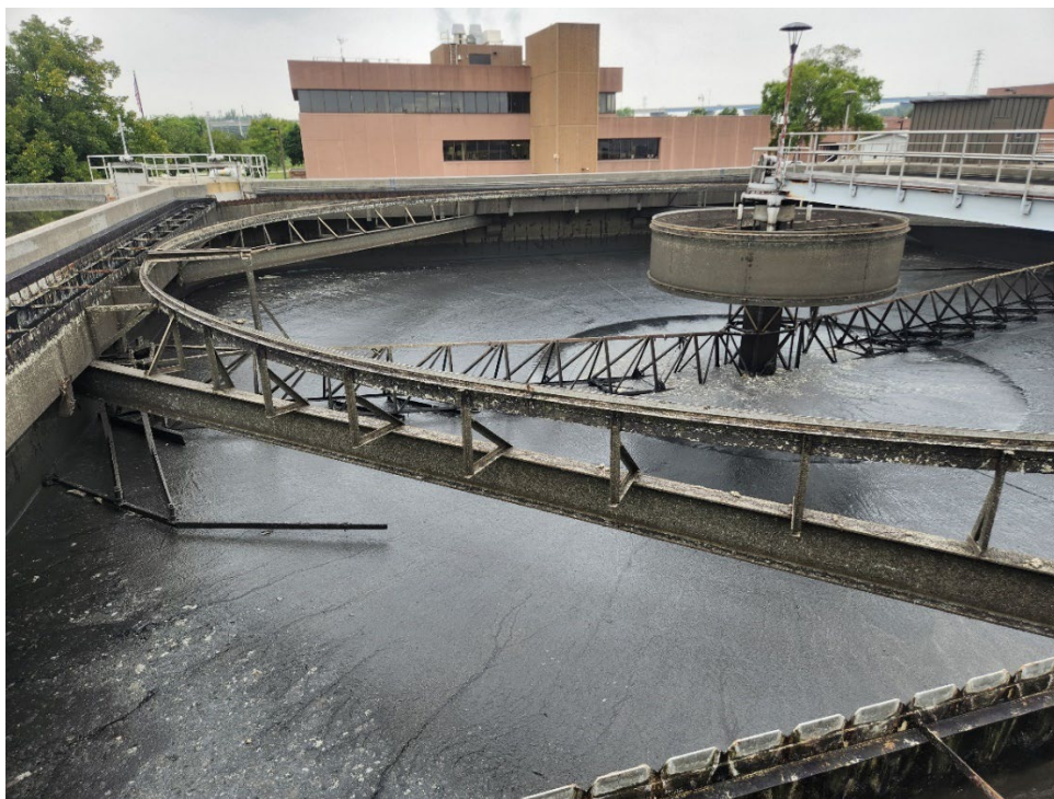
LAST CLARIFIER (PC #4) DRAINED AND PREPPED FOR DEMO
