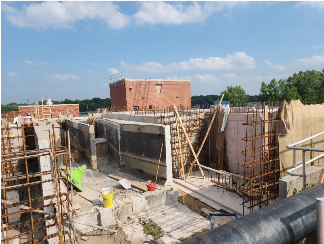
CONCRETE CONSTRUCTION OF GRIT TANKS AND CHANNELS
