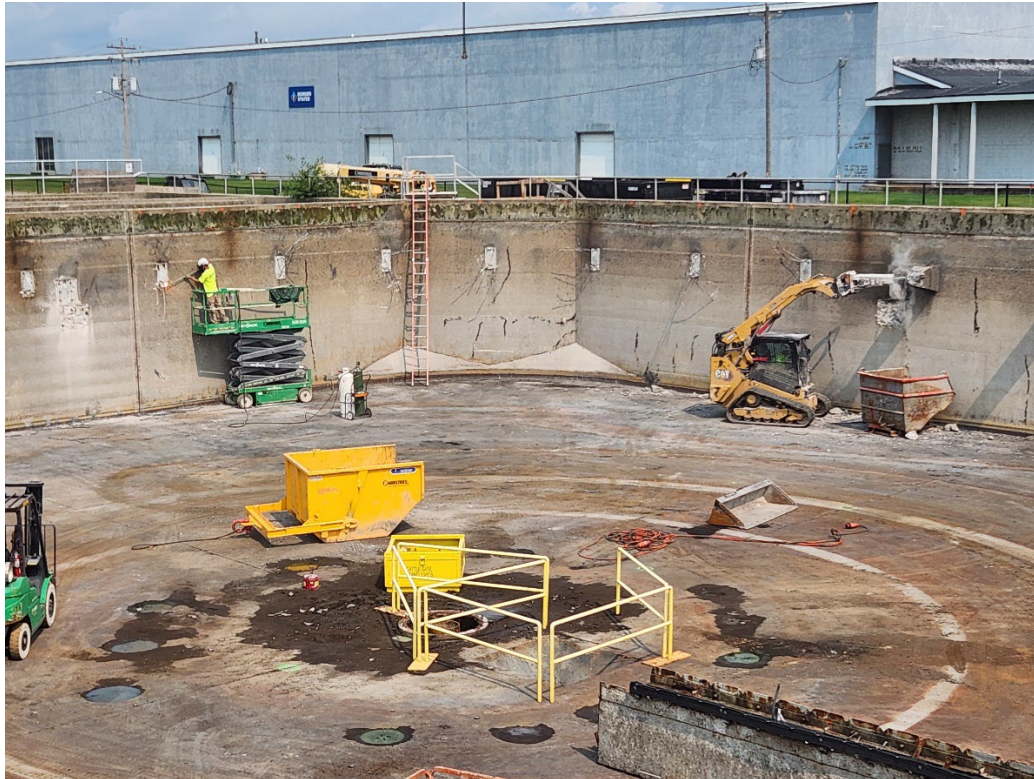
DEMOLITION AND WALL PREP IN FC #4
