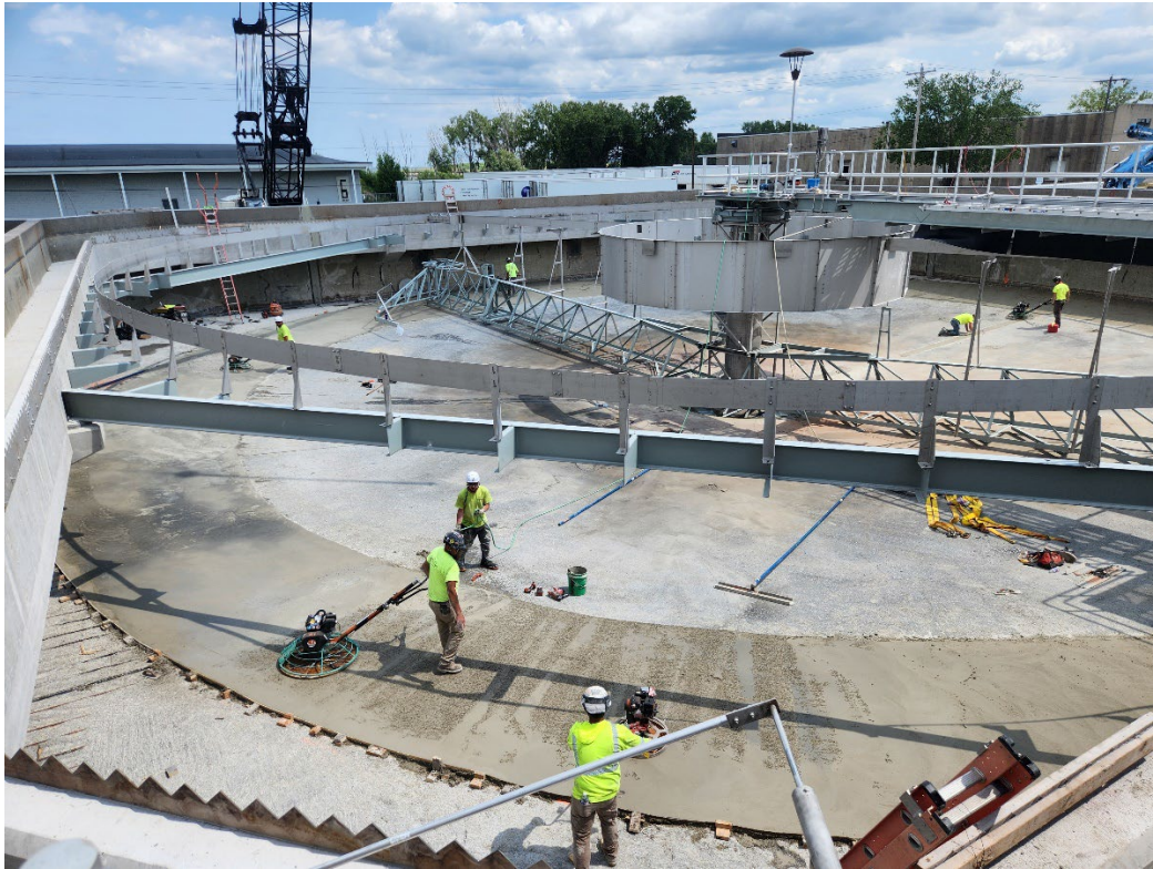
CONCRETE FLOOR REPAIR IN PC #1
