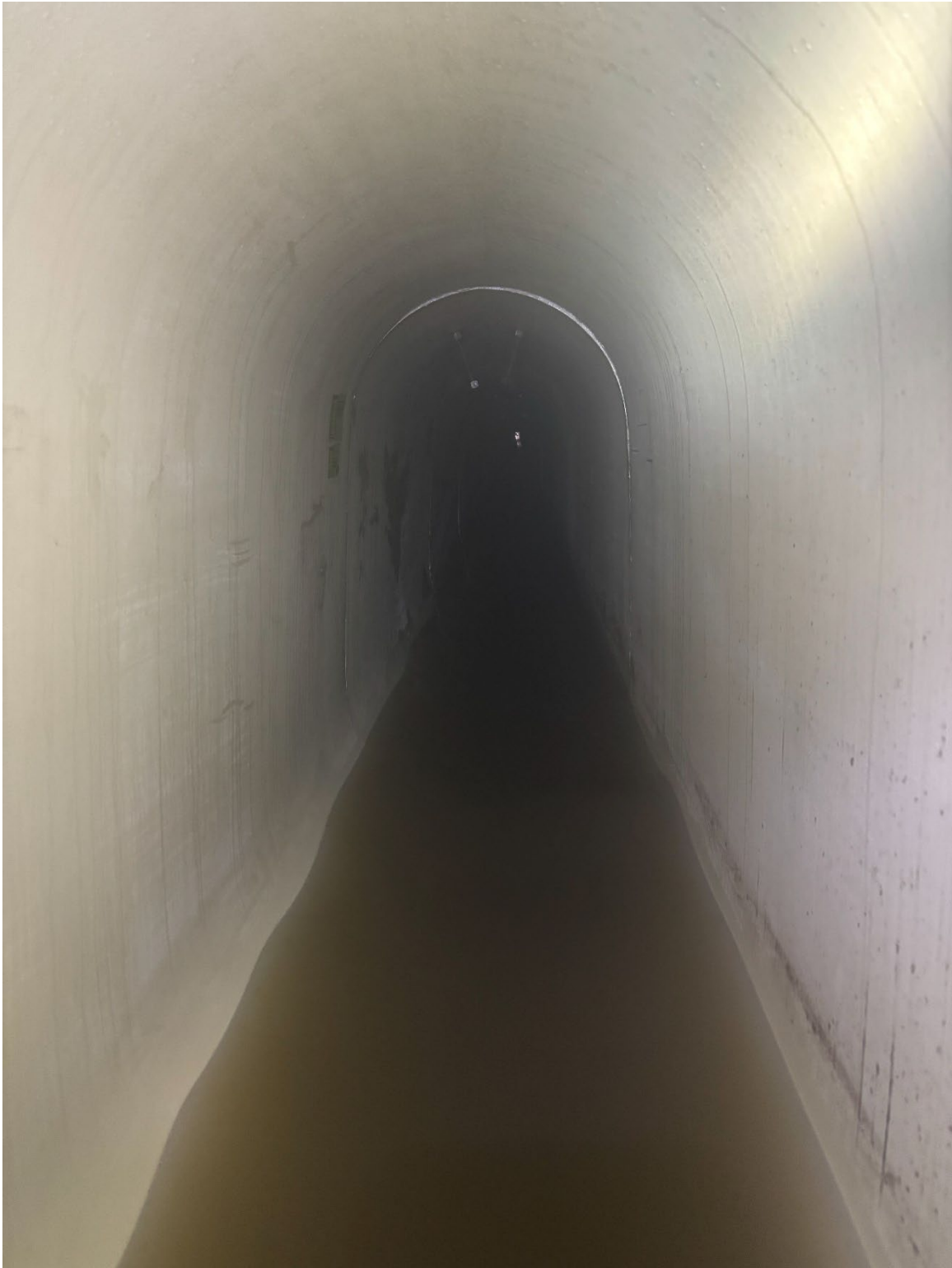
Photo 1 – Inside the 48-inch FRP pipe installed in the East Fox River Interceptor.
