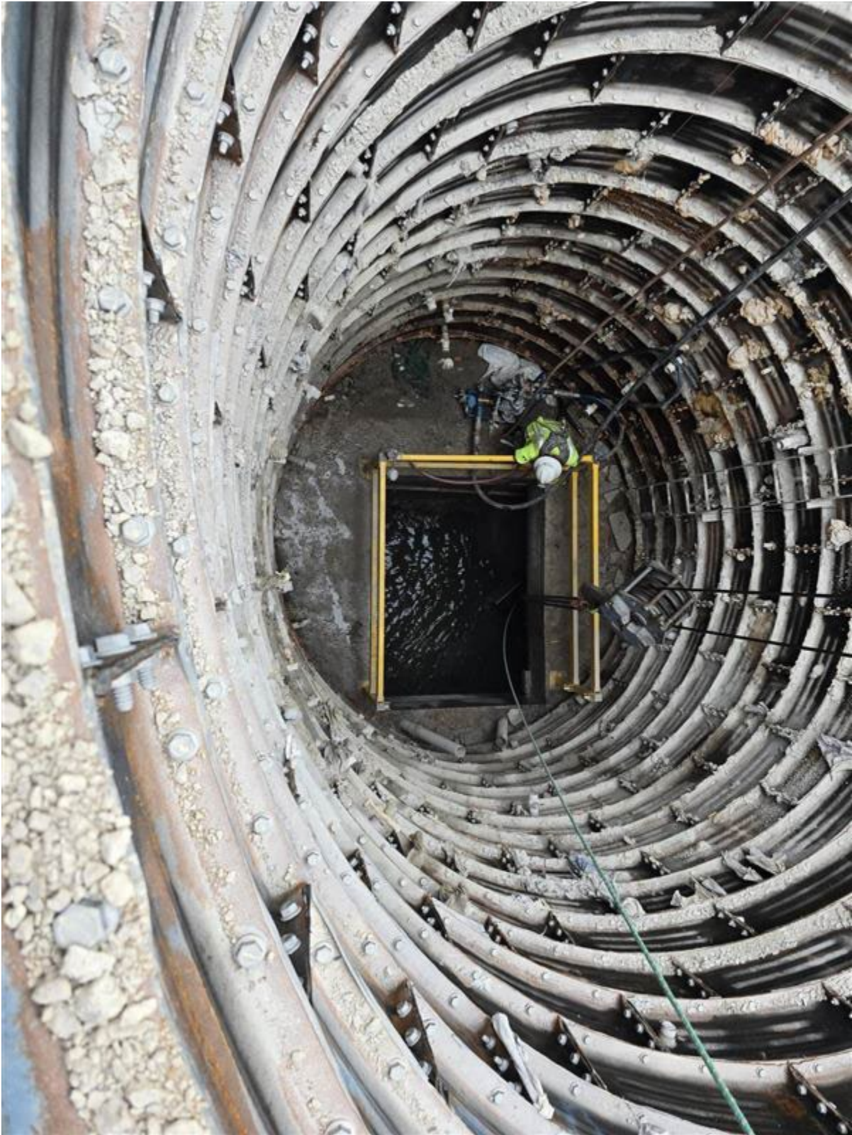
Photo 2 – Main Street Access Pit after excavation and concrete removal.
