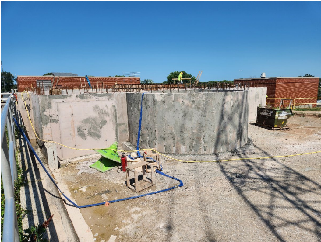
GRIT TANK #2 NEARING COMPLETION
