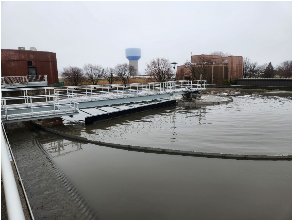
REHABILITATED PC #3 AT 7:00 AM ON 4/14/26
