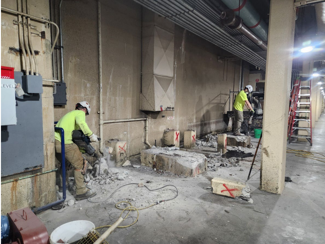
DEMOLITION OF OLD SLUDGE PUMP BASES IN TUNNEL A
