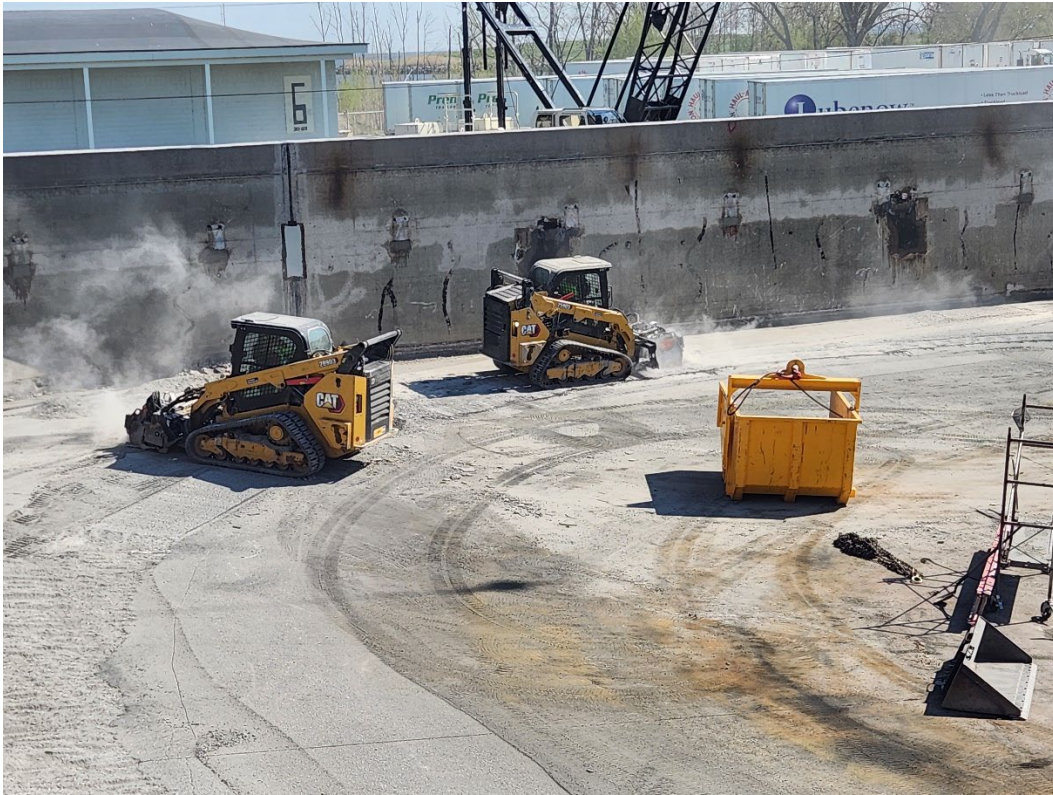
GRINDING DEFECTIVE CONCRETE BASE MATERIAL IN PC #1
