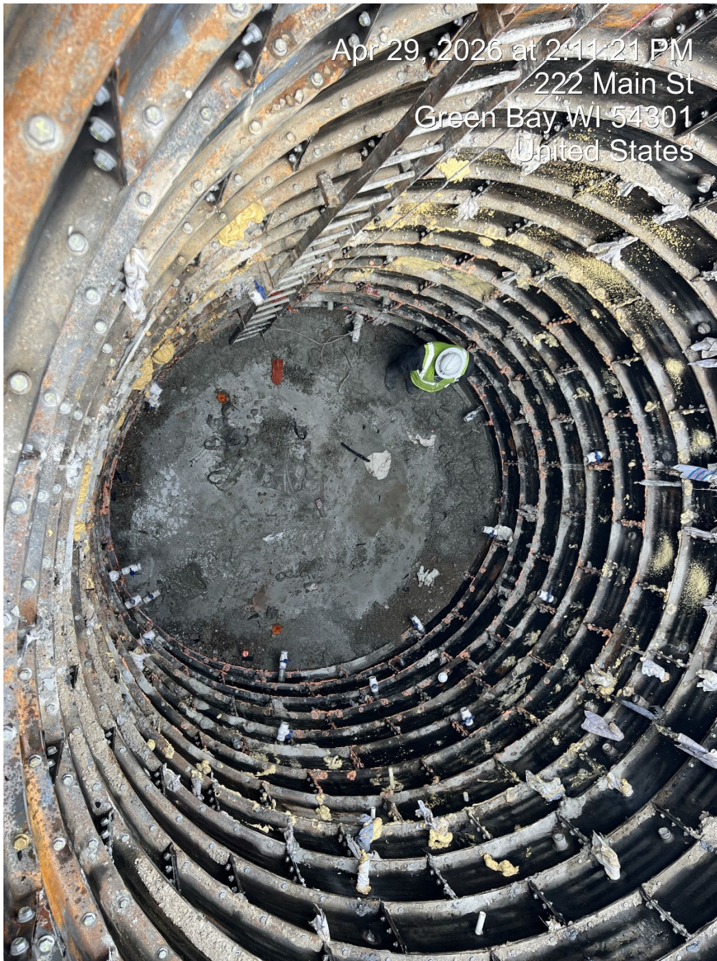
Photo 3 – Main Street Access Pit after excavation was completed.
