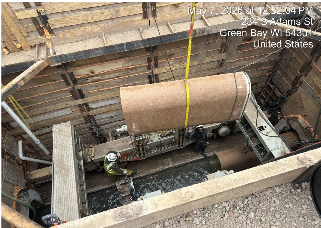
Photo 2 – 42-inch FRP pipe installation into EFR interceptor.
