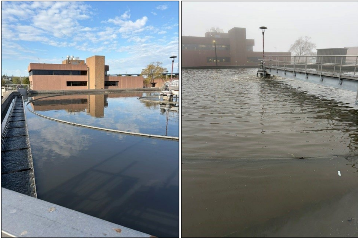
GBF Primary Clarifier 4 Operations: Normal Operation Compared to April High Flow Conditions
