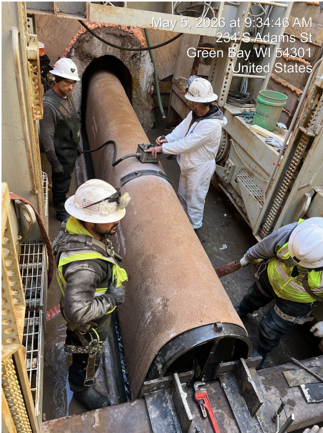
Photo 3 – 42-inch FRP pipe installation into EFR interceptor.
