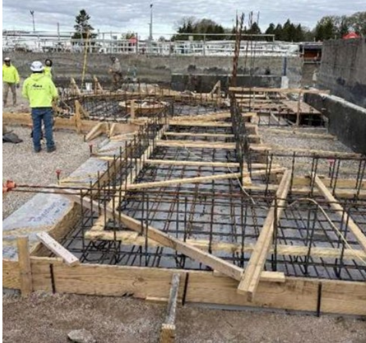
Figure 1: Progress on framing and pouring the new grit removal tanks.
