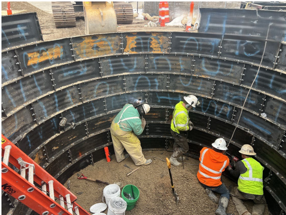
Photo 3 – Construction of the Main Street access pit.
