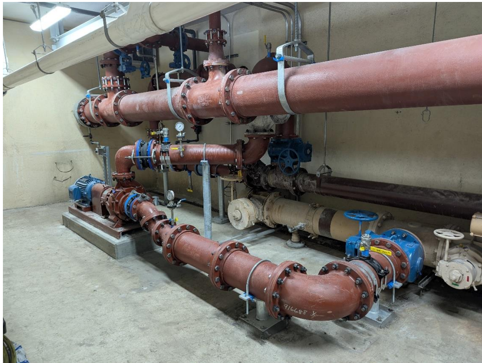
Figure 2: New Sludge Feed Pump Installation
