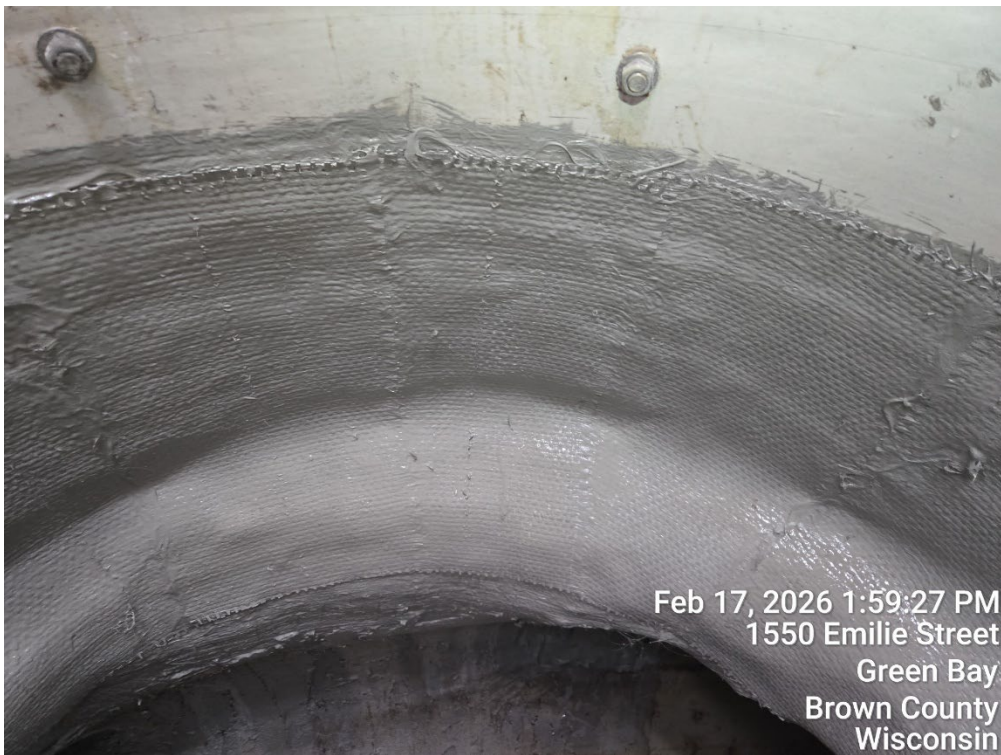
Photo 2 – Manhole rehabilitation including new insert, interior coating, and fiberglass laminations.
