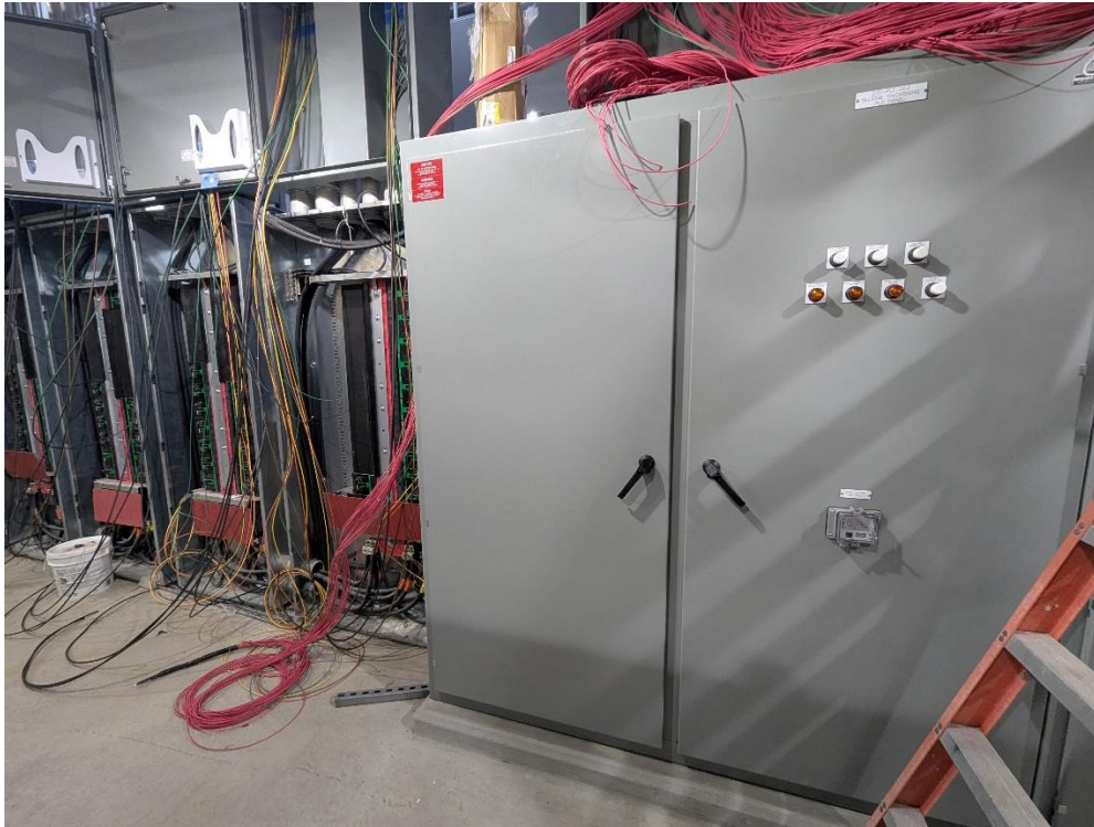
Figure 1: Wiring in Progress of Control and Power Panels
