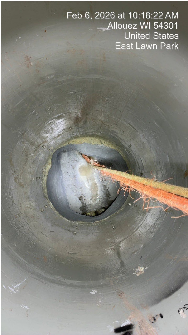
Photo 3 – Manhole rehabilitation including new insert, interior coating, and fiberglass laminations.
