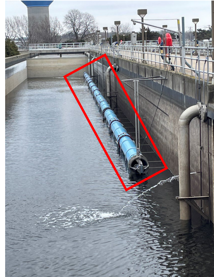
Mixed Liquor Recycle Pump
