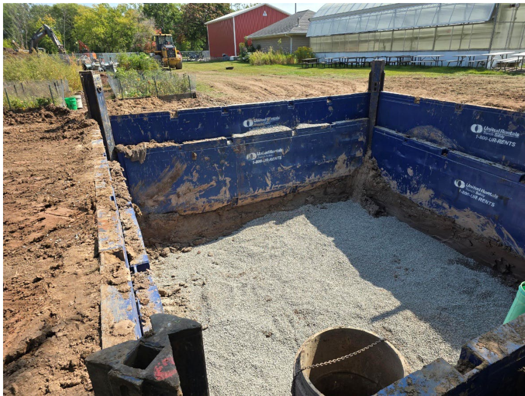
Photo 2 – Contractor excavating pit to set temporary conveyance pumps.
