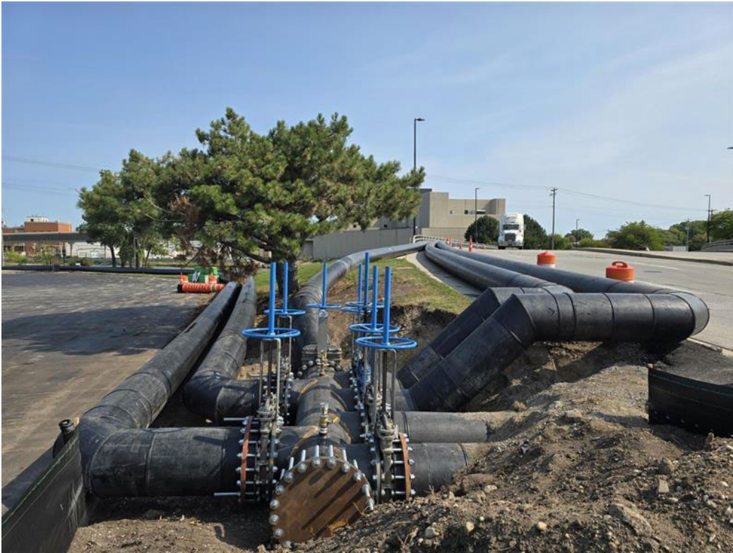
Photo 1 – Temporary conveyance junction on the northwest side of N Monroe Avenue.
