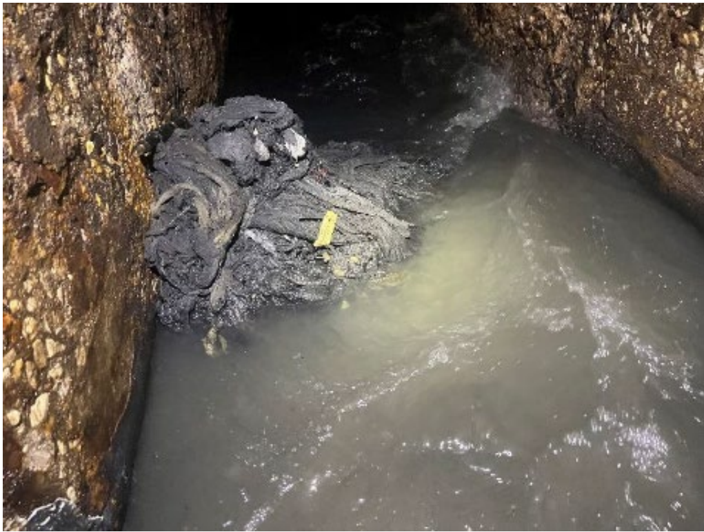
Photo 1 – Rag ball removed from the EFR interceptor.
