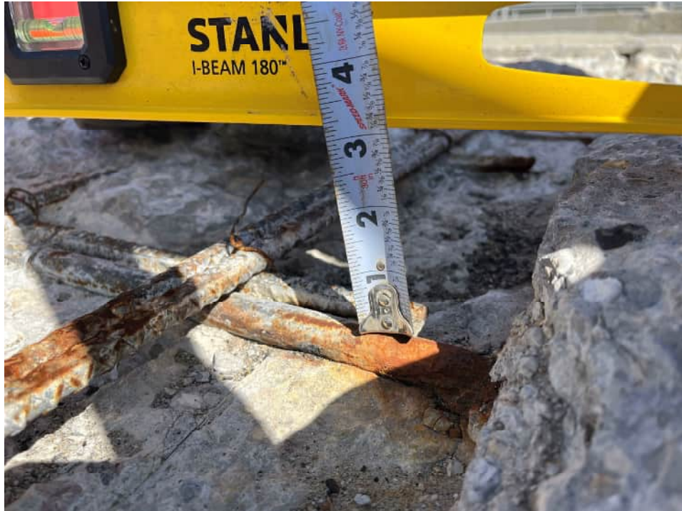
Existing Doweled Connection
