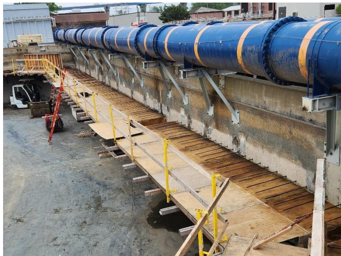
FINAL CLARIFIER #6 – PIPE SUPPORT MODIFICATIONS AND LAUNDER FORMING
