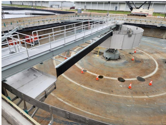
FINAL CLARIFIER #1 – STRUCTURAL AND MECHANICAL NEARLY COMPLETE
