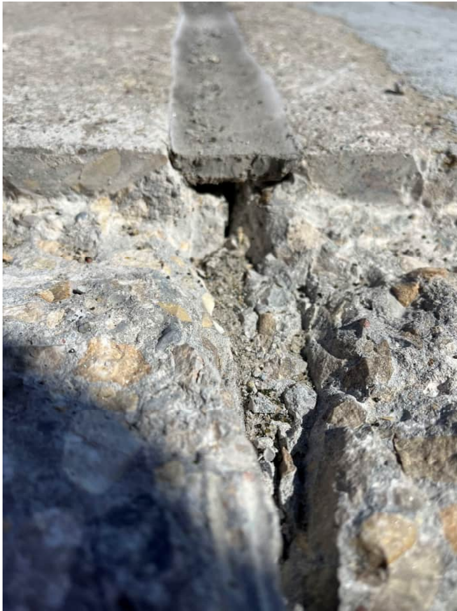
Existing Construction Joint
