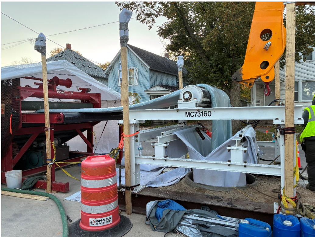
Photo 1 – Michels preparing for the first install of 48" CIPP Liner.
