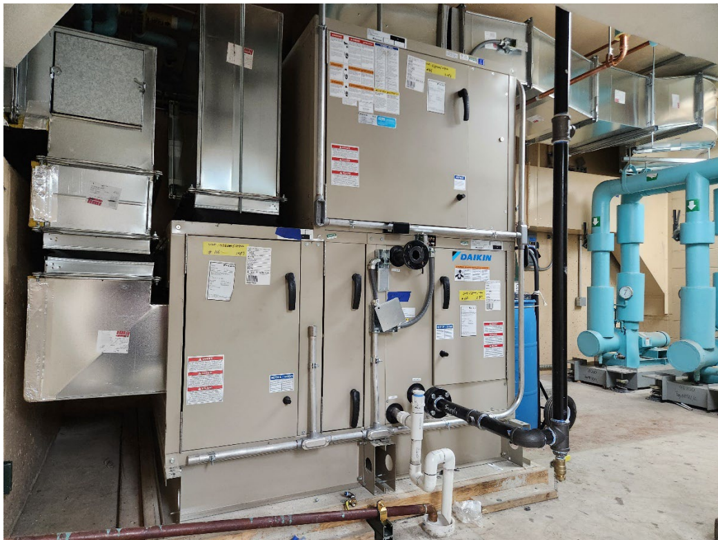
NEW AIR HANDLING UNIT A-10 SERVING BASEMENT ELECTRICAL ROOMS
