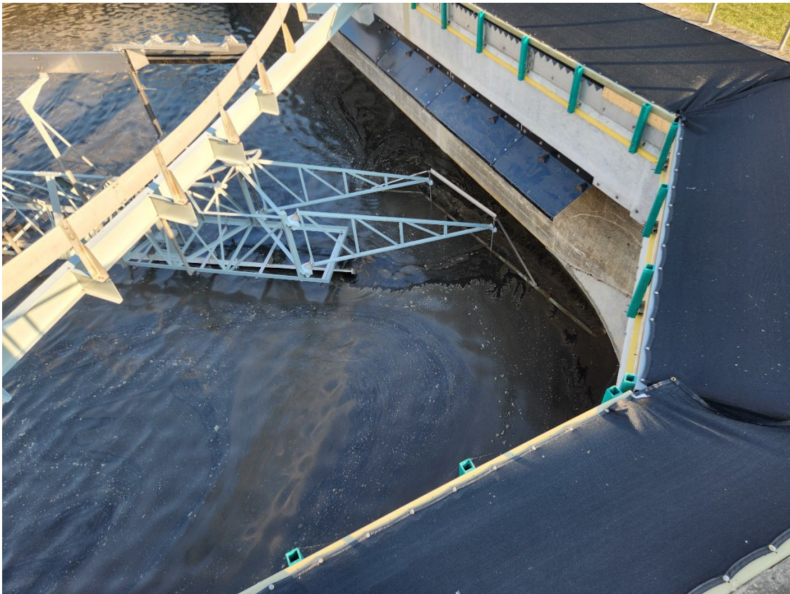
TRACKING DEPLOYMENT OF CORNER SWEEP WHILE FILLING FC1
