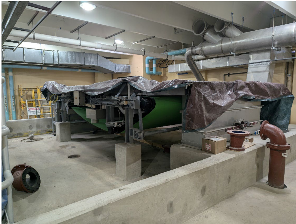
Figure 1: New Gravity Belt Thickener in the Process of being Installed
