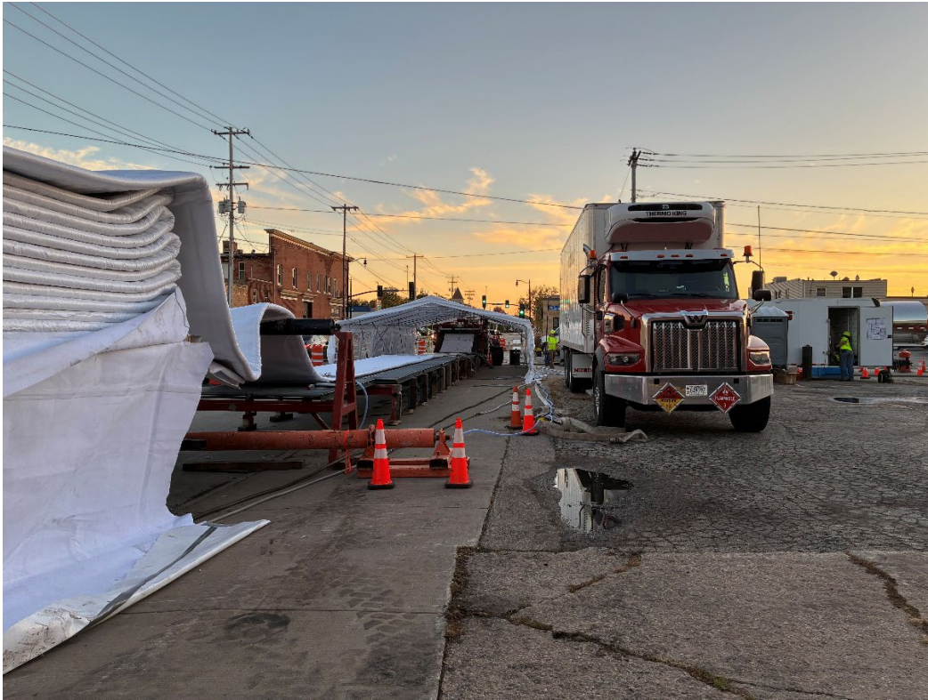
Photo 1 – Michels preparing for the first install of 48" CIPP Liner.
