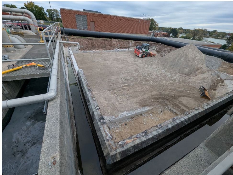
Figure 2: Temporary Bypass Piping and Preliminary Treatment Unit Demolition
