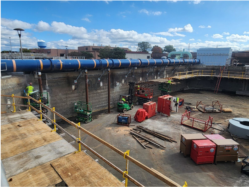
TEMPORARY PIPE SUPPORTS (LT) AND NEW BRACES (RT) FOR FC7 WCD #20
