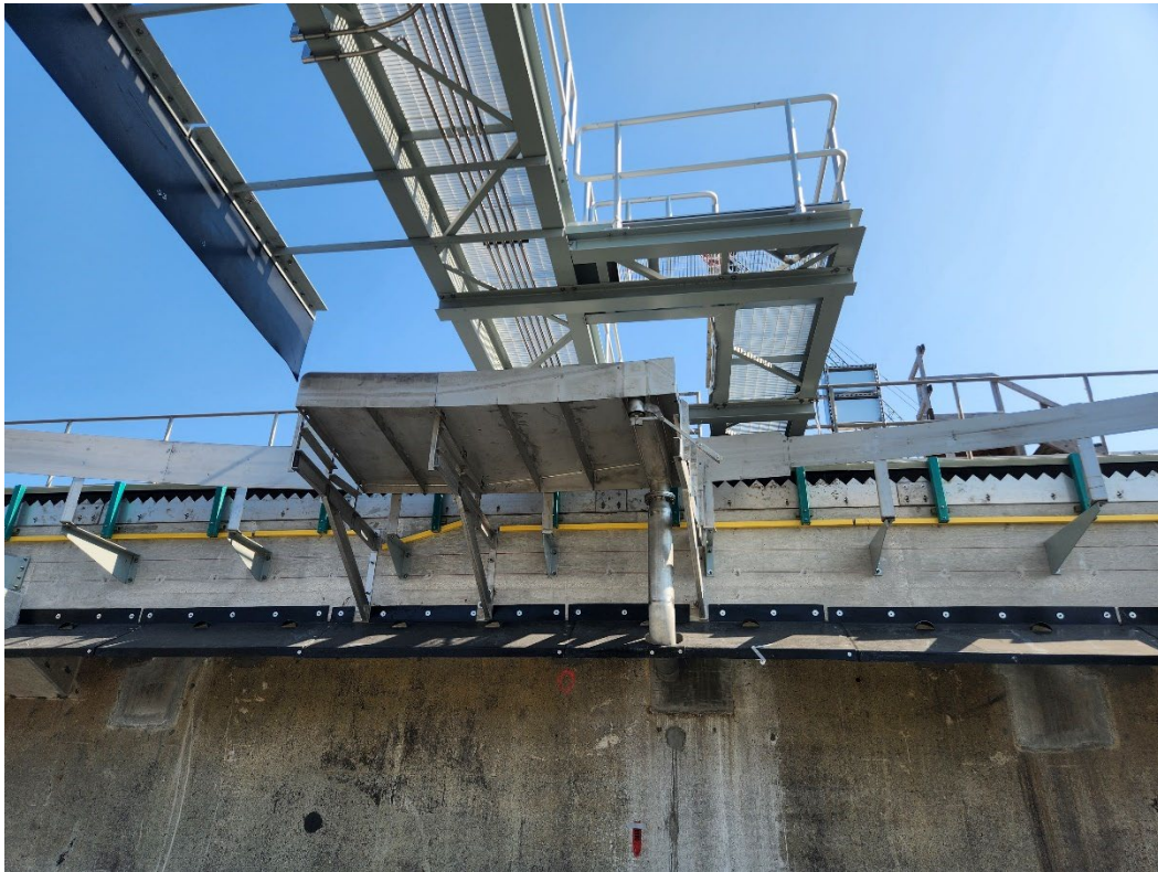
SCUM BEACH AND ANTI-ROTATION Baffle FROM UNDERNEATH BRIDGE
