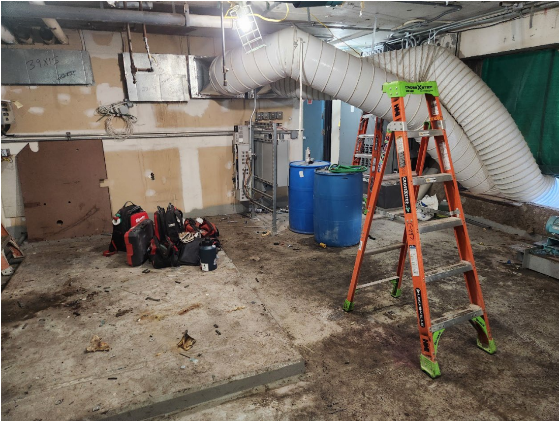
SOUTH ROOFTOP MECHANICAL ROOM DEMO WITH TEMP COOLING TO DATA CENTER
