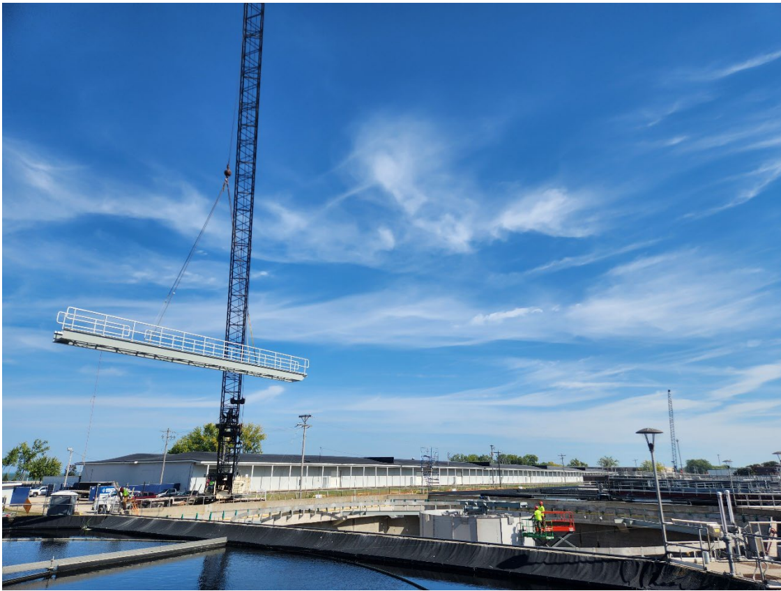
PLACING BRIDGE FOR FC3
