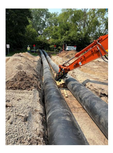
Photo 2 – Contractor burying the temporary conveyance piping at the N Irwin Street crossing.
