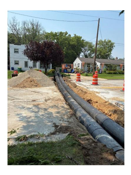
Photo 1 – Contractor burying the temporary conveyance piping at the N Baird Street crossing.
