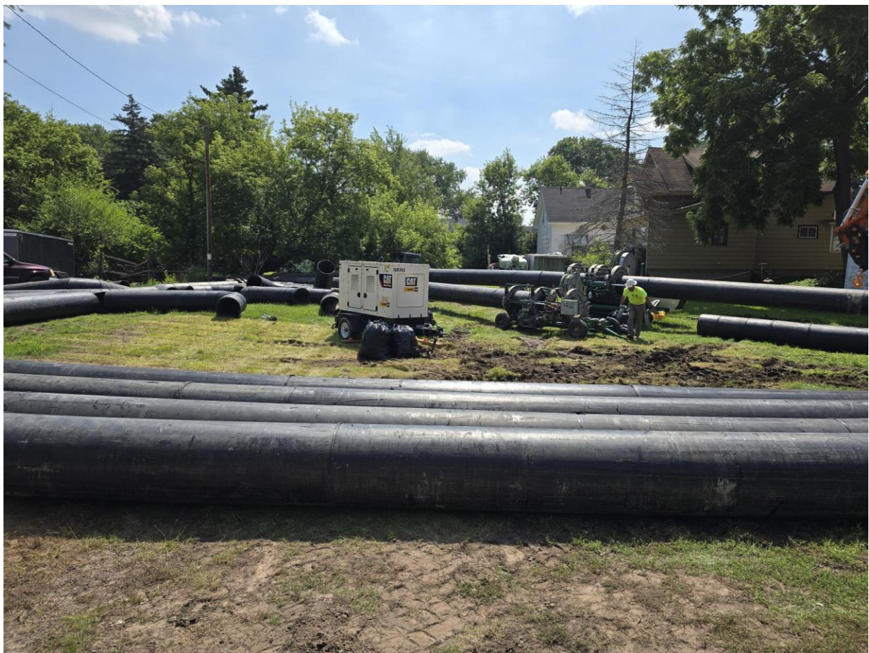
Photo 1 – Equipment and HDPE pipe being delivered and staged for bypass setup.
