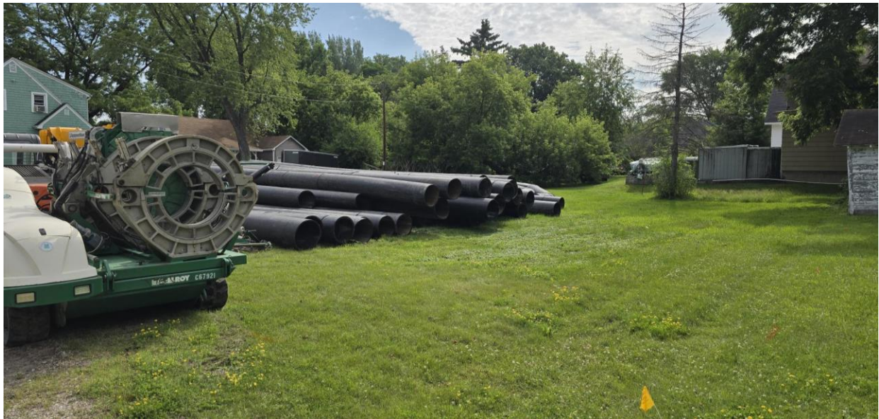
Photo 1 – Equipment and HDPE pipe being delivered and staged for bypass setup.
