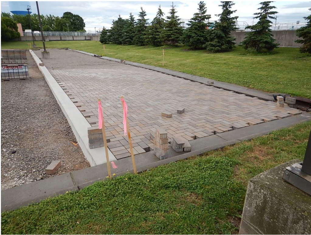
Photo 1 – Placement of the permeable pavers
