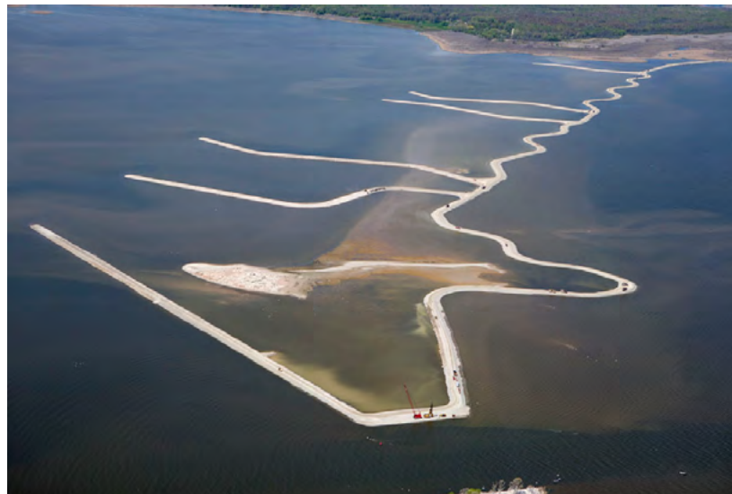
Figure 91: Cat Island spine construction, May 2013.
