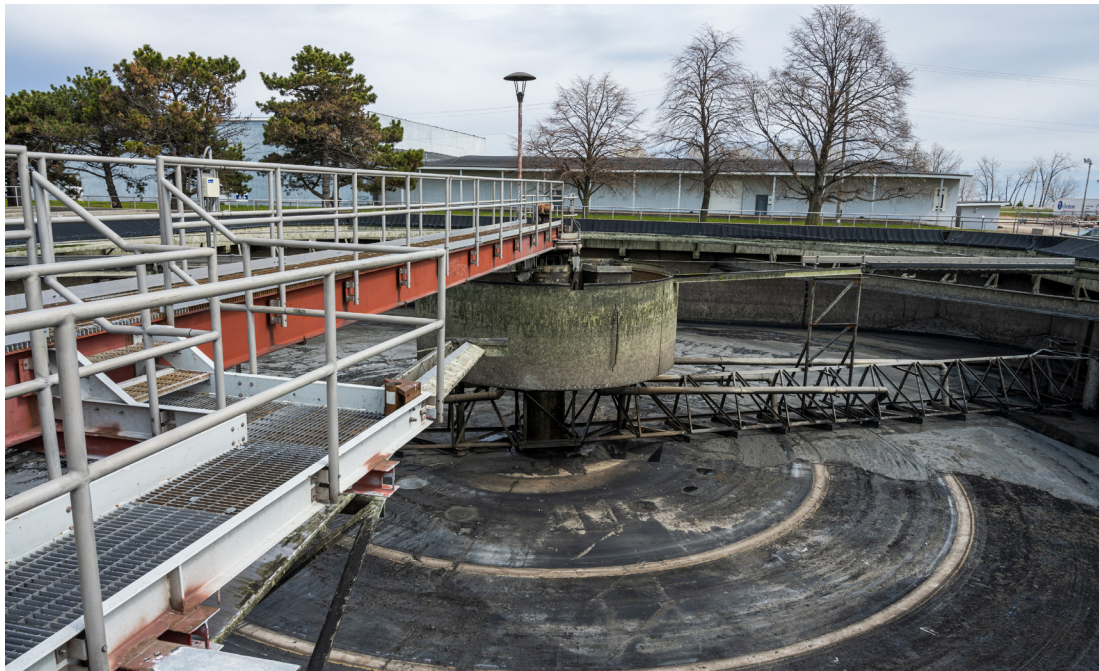
Image captions: Aging clarifier and equipment in need of replacement.
